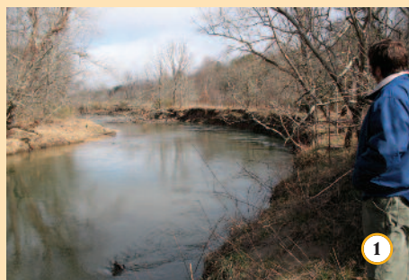
Bank stabilization project at Tessentee Creek Preserve. The rock vane protects the bank from shear stress. The banks were sloped to create a bench, matted with biodegradable coir fabric, live-staked and planted with native seedlings and a native riparian mixture. The stone steps allow boaters to access the creek.
